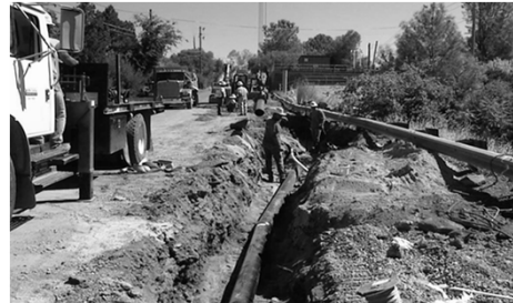
Installation of Waterline In Placer County
