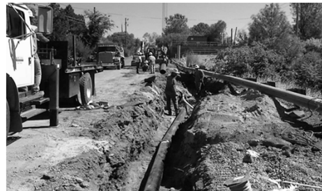
Installation of new water system in Placer County, included installation of private laterals for low income households.
