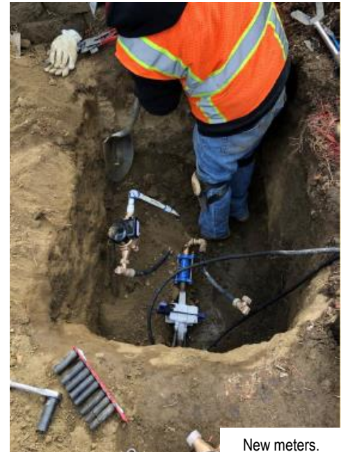
New water line.
