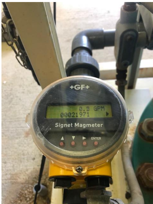
New Backwash Flow Meter
