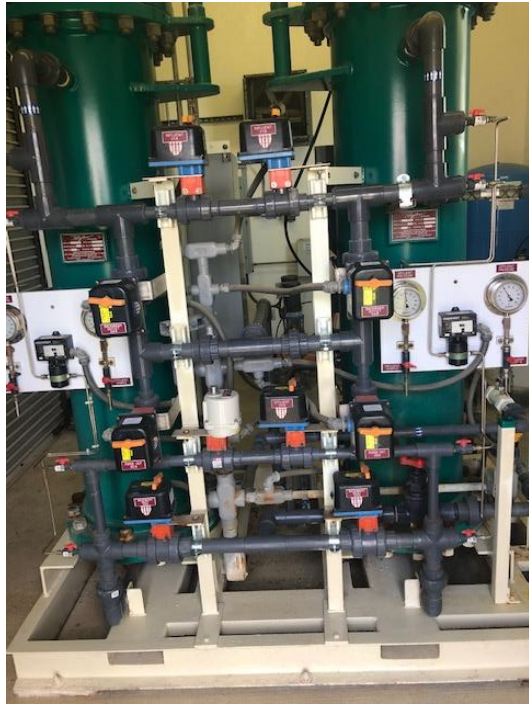
Re-piped Influent and Effluent
